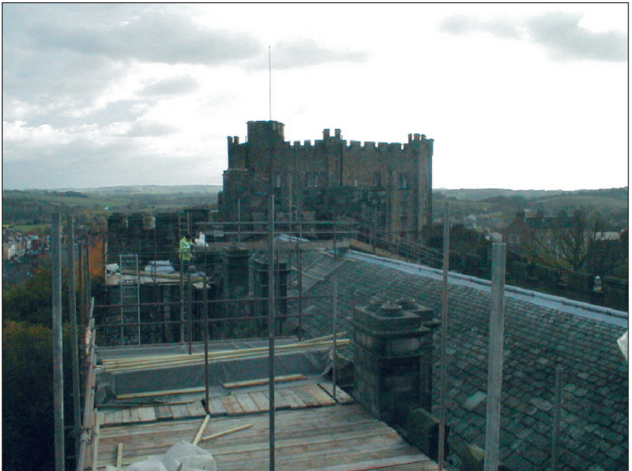
Restoration work is now proceeding on the Castle roof.
